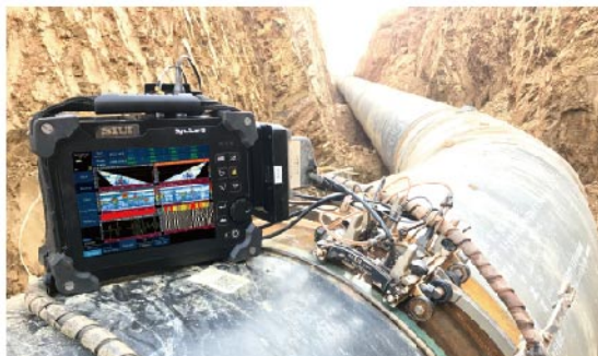
Pipe weld inspection
