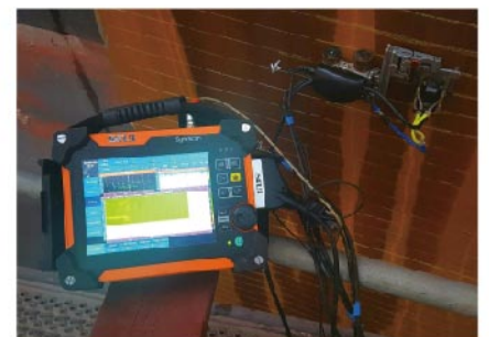
PA corrosion solution
