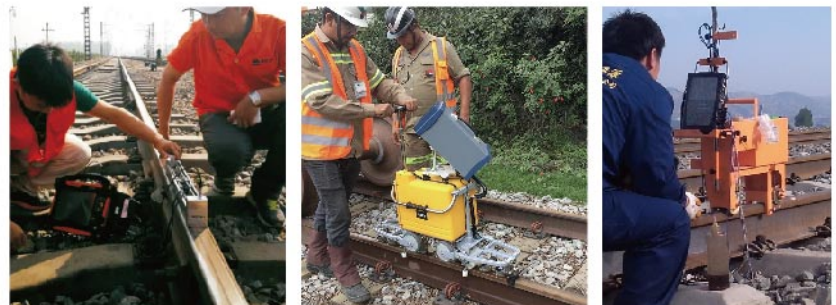
● PA testing for weld
